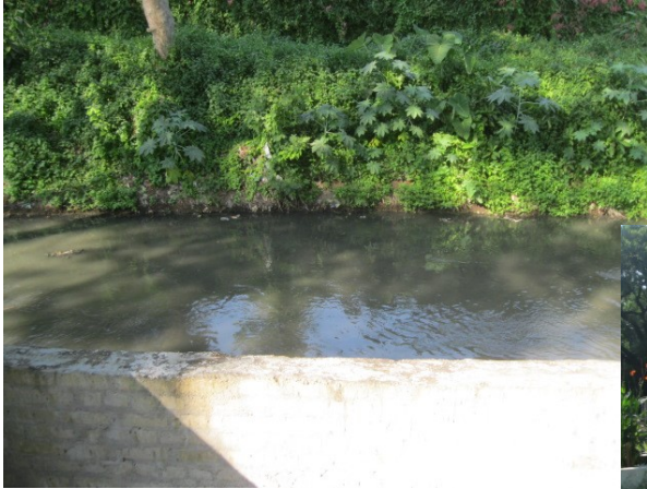
Raw sewage in nallah
